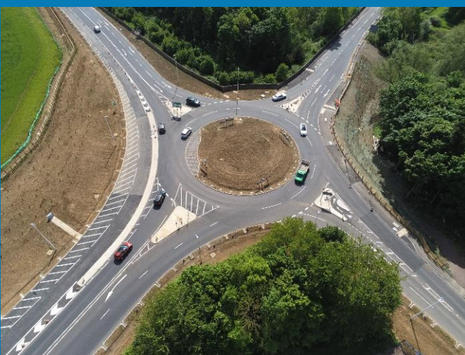
A602 roundabout at completion
