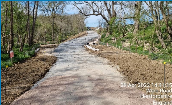
Cycle track construction progress
