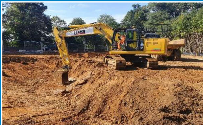
Excavation of drainage attenuation pond opposite Heath Mount School
